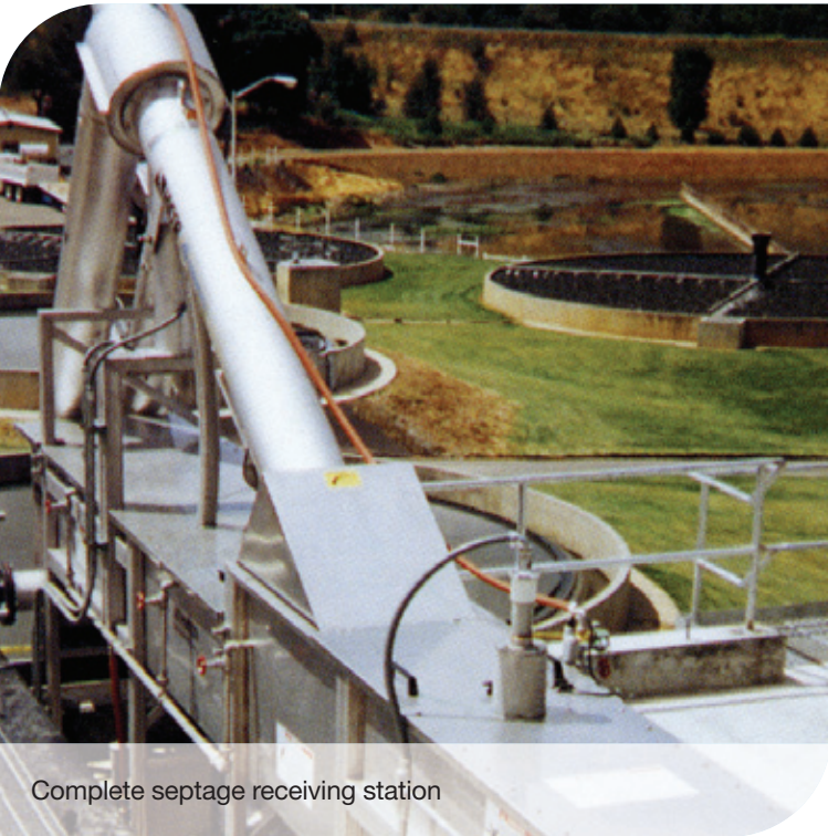
The Combi ® System automatically screens and degrits septage
